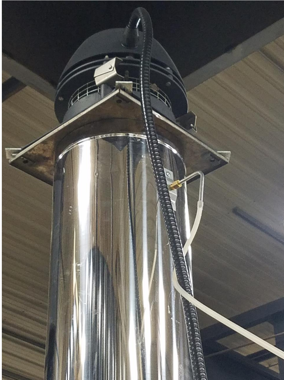
Picture 4 – Blaze 6 I/O Flue Vent Pipe with Chimney Fan Component
