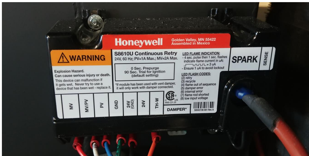
Picture 11 – Blaze 6 I/O Pilot Ignition Module Component
