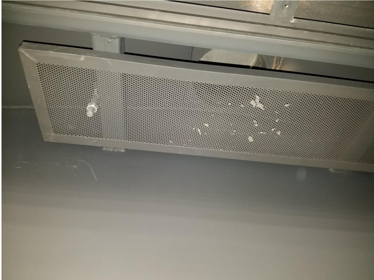
Picture 5 – Blaze 6 I/O Non-Load-Bearing Flue Gas Baffle
