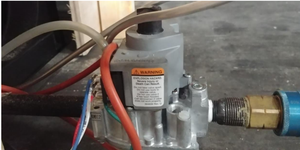
Picture 12 – Blaze 6 I/O Automatic Gas Valve Component
