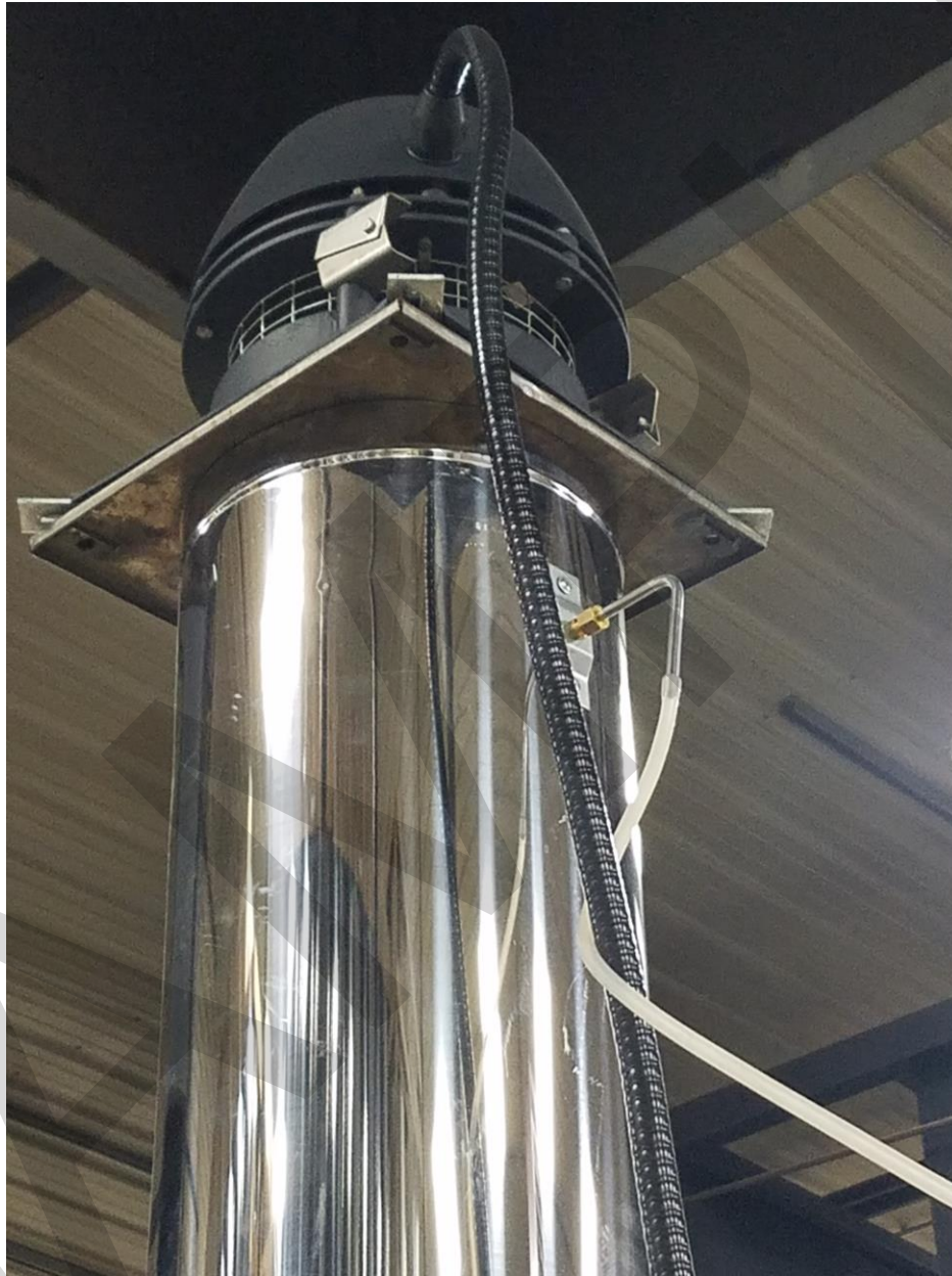
Picture 4 – Blaze 6 Flue Vent Pipe with Chimney Fan Component
