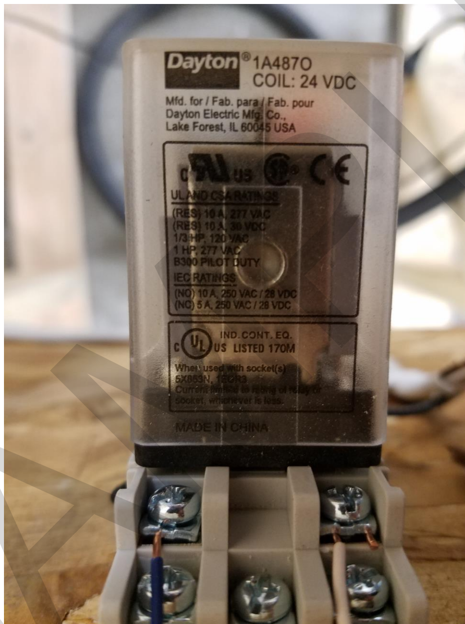
Picture 11 – Blaze 6 Electrical Relay Component
