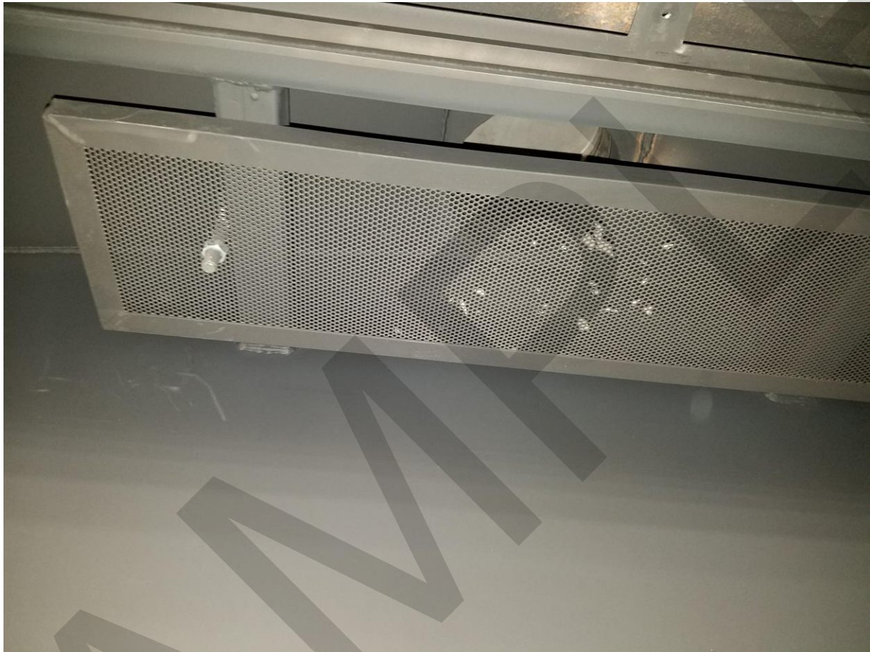
Picture 5 – Blaze 6 Non-Load-Bearing Flue Gas Baffle
