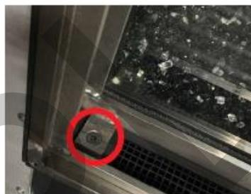
Step 1: Install inner pane of glass in the channel
