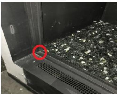
Step 3: Install the outer glass in the channel
