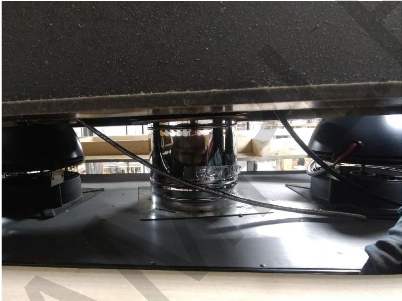
Picture 9 – Model 8’ See-Through Fireplace with Logs Dual Heat Reliefs and Single Flue (Top of Appliance)
