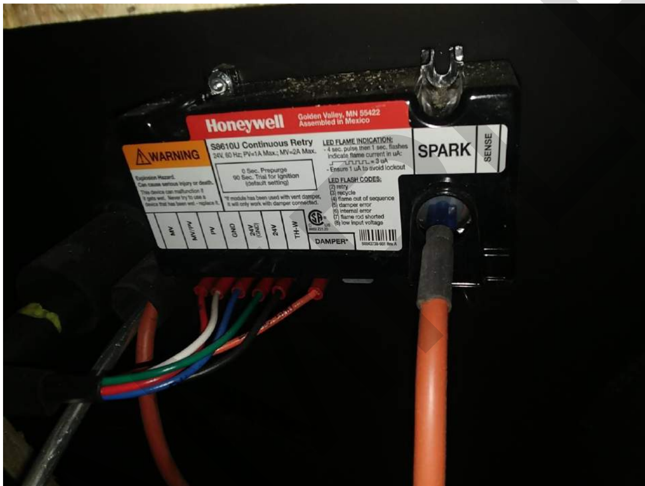
Picture 7 – Model 8’ See-Through Fireplace with Logs Pilot Ignition Module Component
