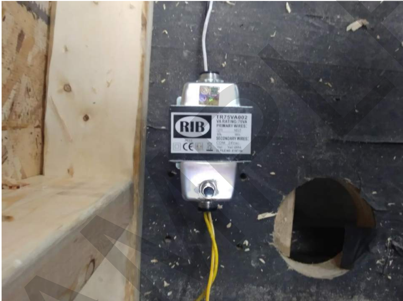
Picture 8 – Model 8’ See-Through Fireplace with Logs Transformer Component
