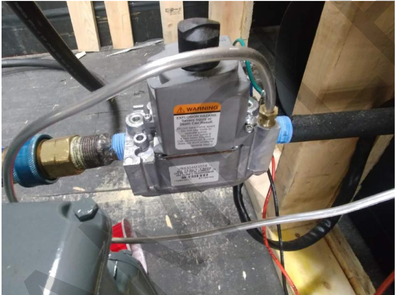
Picture 10 – Model 8’ See-Through Fireplace with Logs Automatic Gas Valve Component
