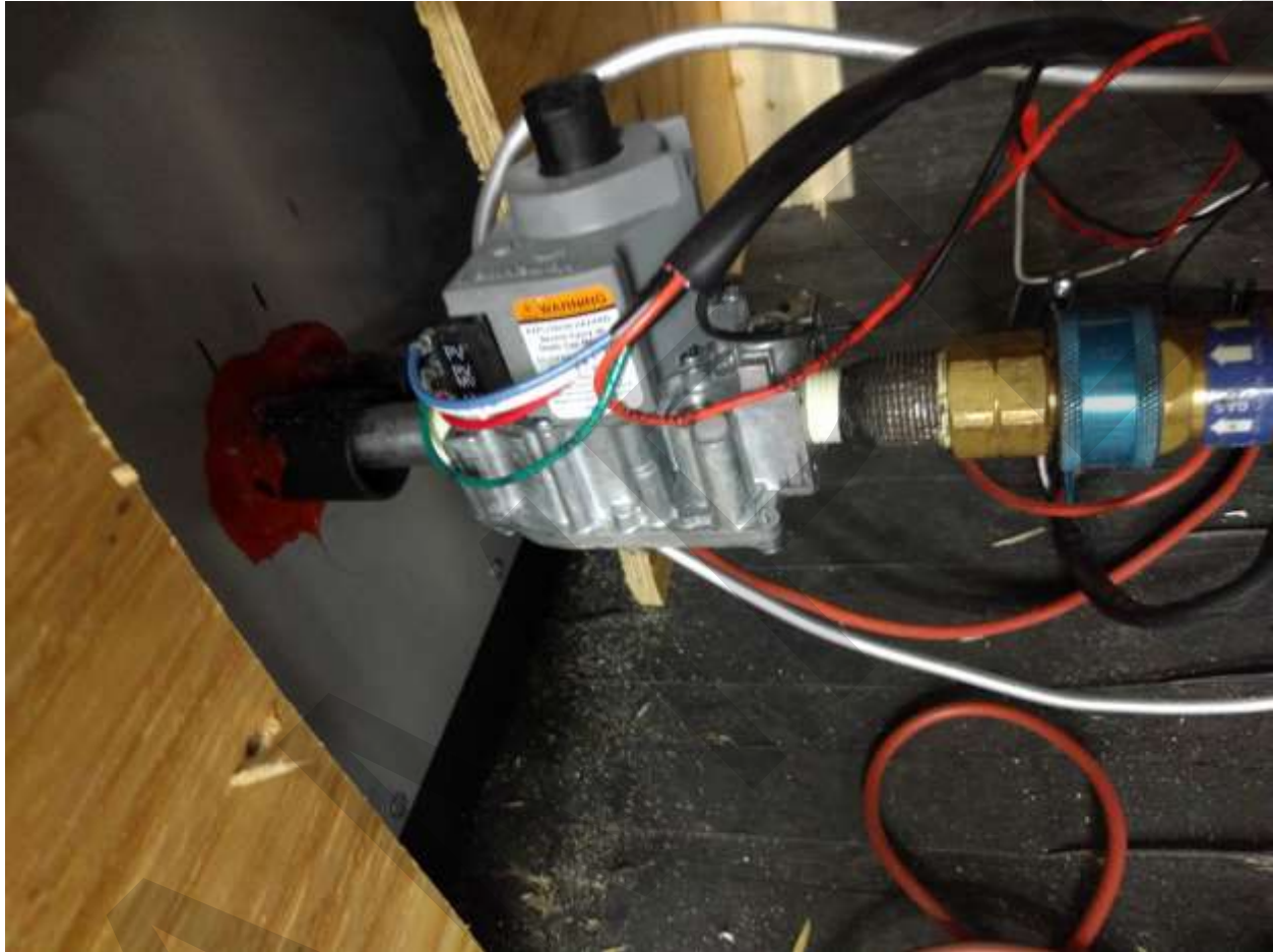
Picture 5 – Linear IO with door Automatic gas valve
