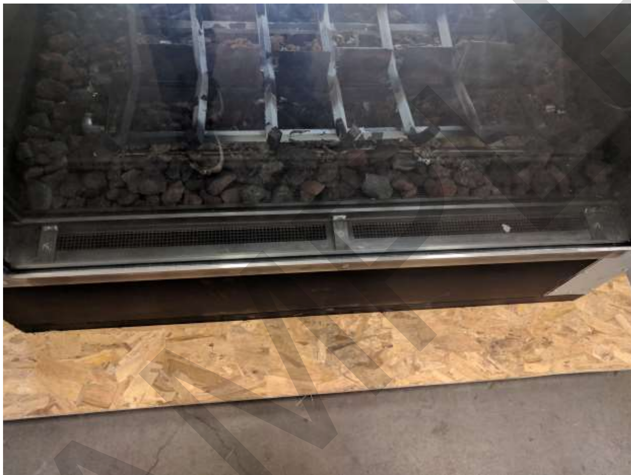
Picture 3 – Linear IO with door View of Dual Pane Glass Front with Glass Cooling Space
