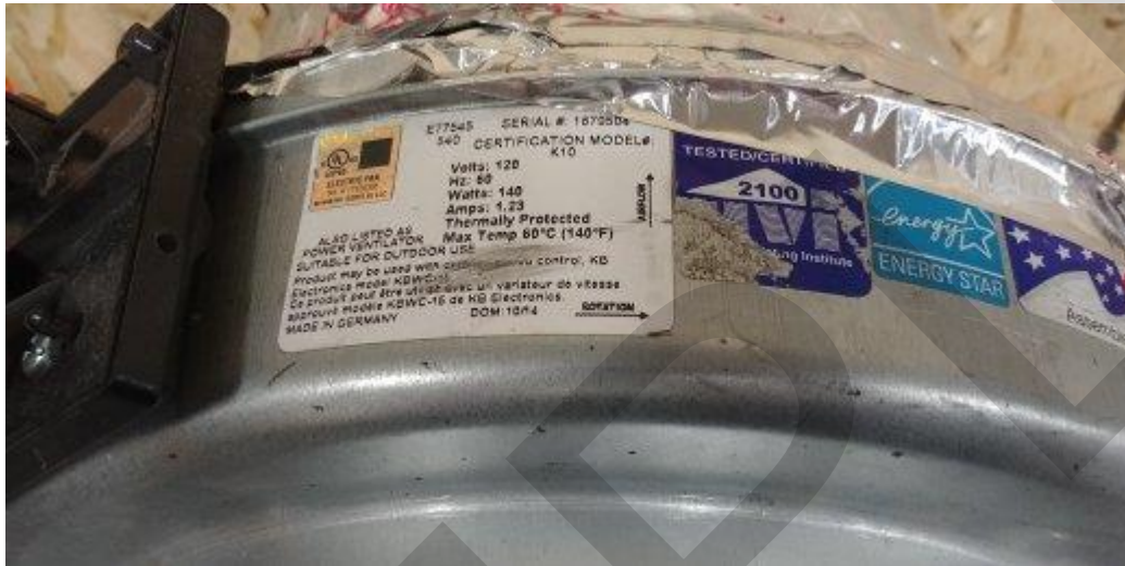
Picture 5 – Single-Sided 7'8" Square Fireplace with Log Set Cooling Air Intake Fan
