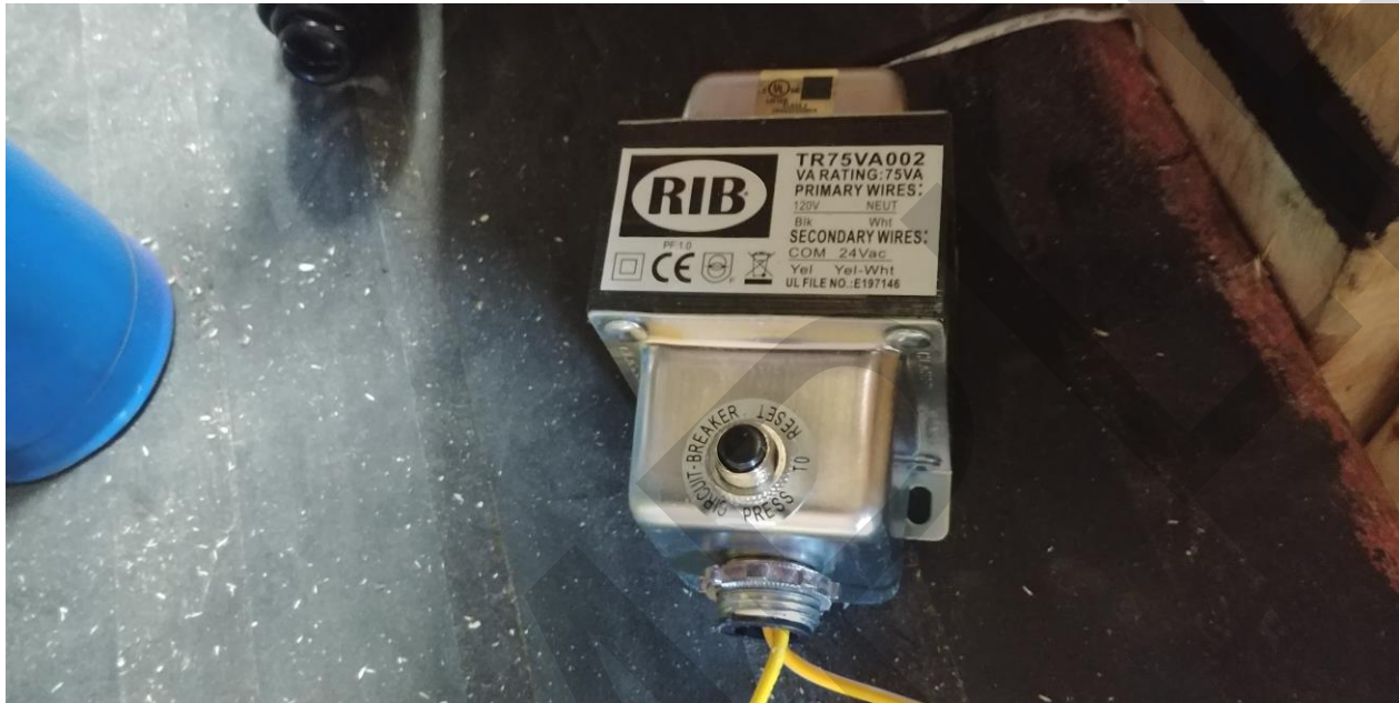
Picture 9 – Custom Gas L-Shaped Fireplace Transformer Component
