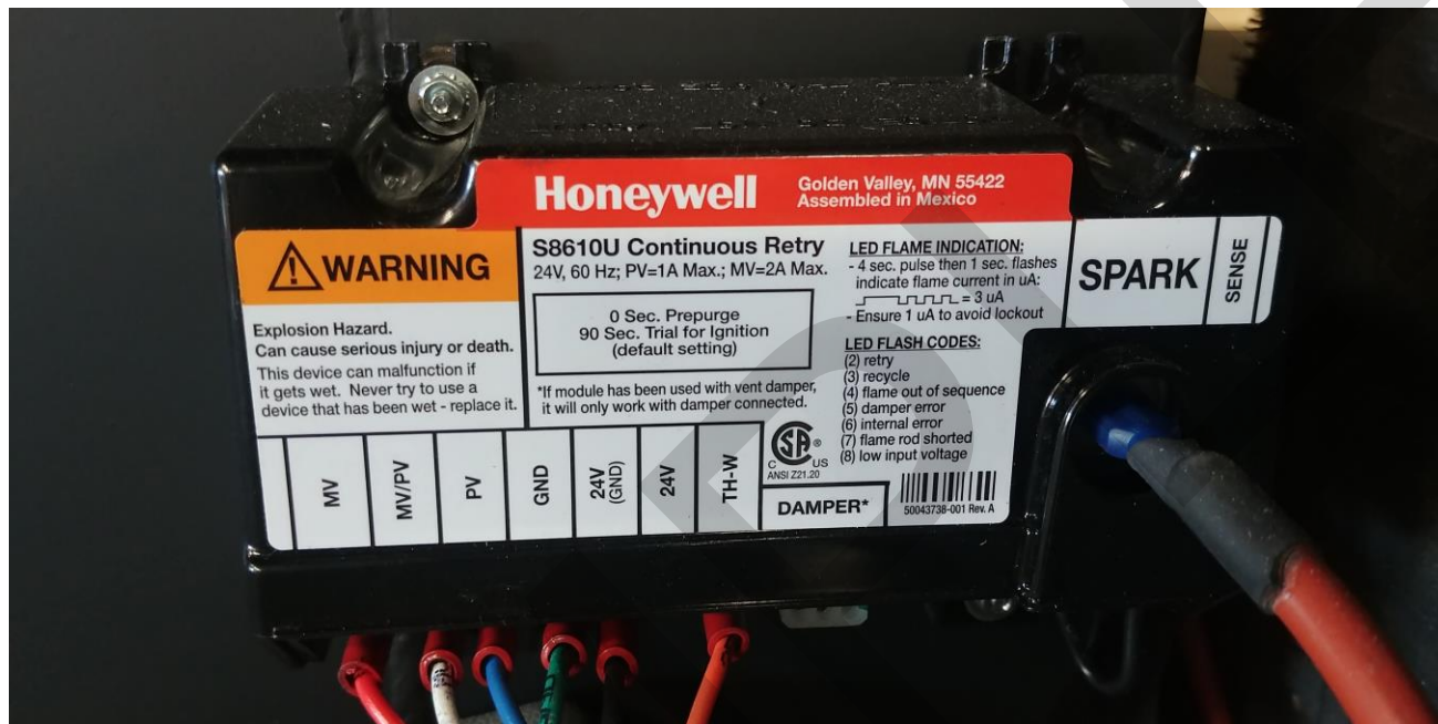
Picture 10 – Custom Gas L-Shaped Fireplace Pilot Ignition Module Component
