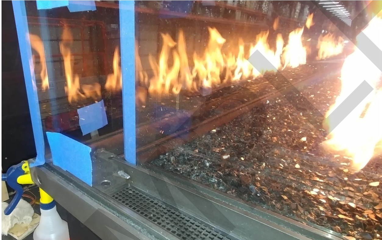
Picture 3 – Custom Gas L-Shaped Fireplace View of Dual Pane Glass with Glass Cooling Space
