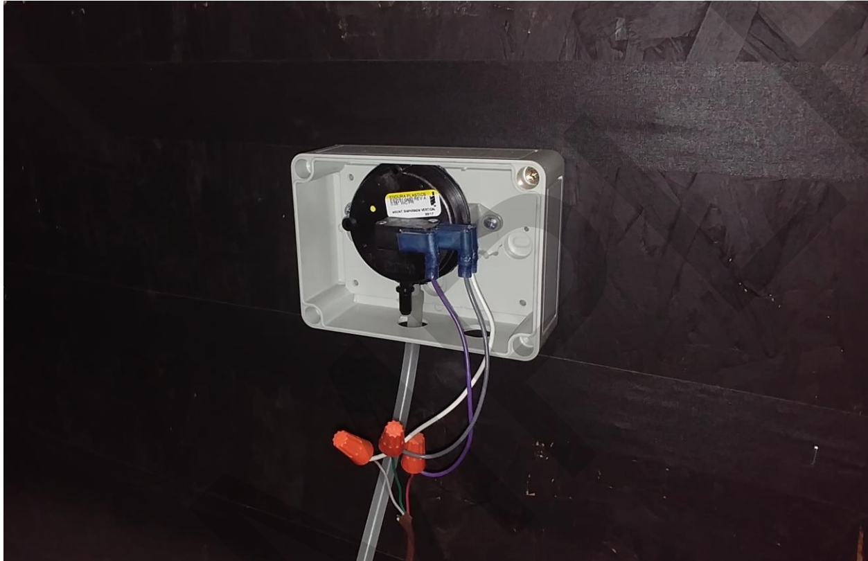
Picture 6 – Custom Gas L-Shaped Fireplace Proven Draft Switch Component
