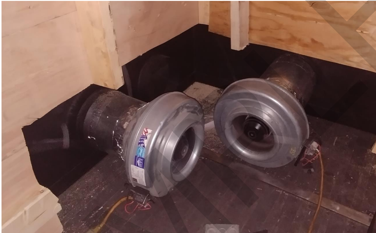
Picture 5 – Custom Gas L-Shaped Fireplace Glass Cooling Air Intake and Combustion Air Intake
