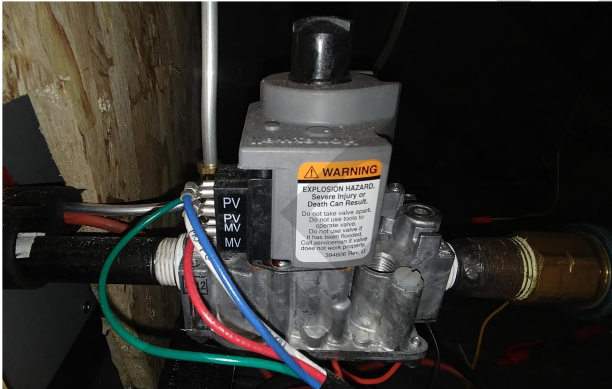
Picture 7 – Custom Gas L-Shaped Fireplace Automatic Gas Valve Component
