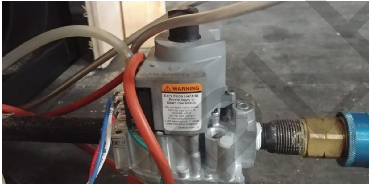
Picture 11 – Custom Gas L-Shaped Fireplace Automatic Gas Valve Component
