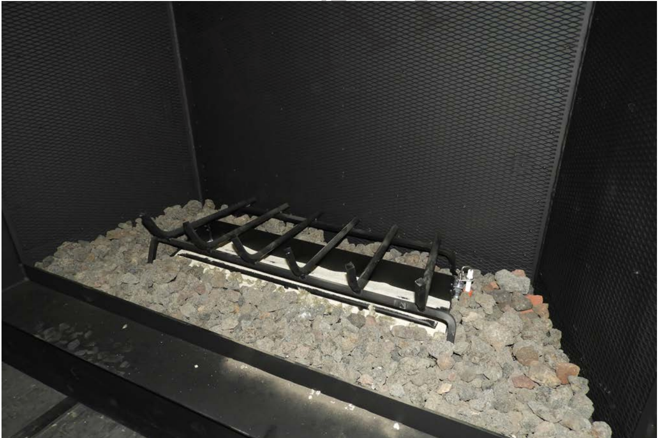
3. Fit grate so legs are snug against the floor of the fireplace.
