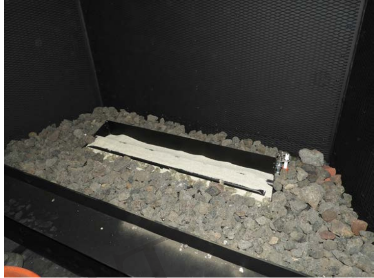
2. Scatter loose lava rocks around bottom of fireplace. Cover front of tray with rocks.
